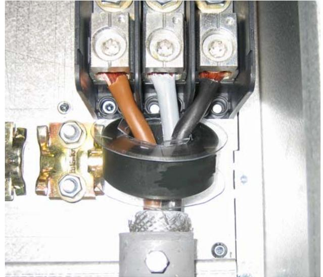
Fig. 49 Ferrite core mounted on the motor cables
