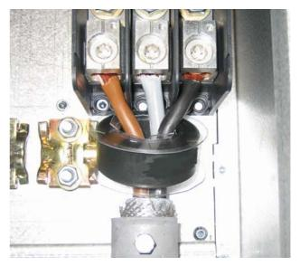
Fig. 49 Ferrite core mounted on the motor cables
